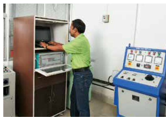
Partial Discharge Test (Digital)
